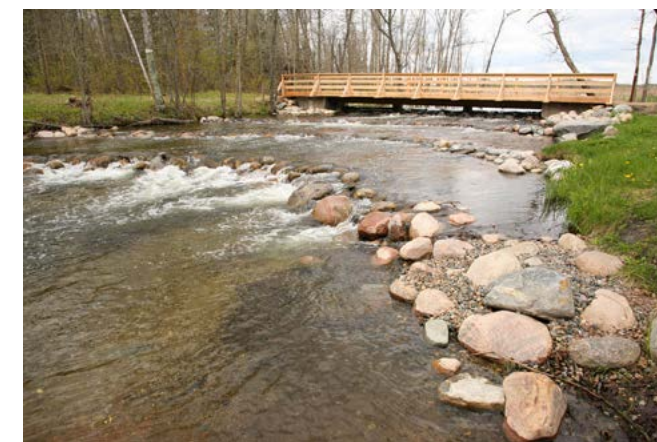
Turtle River Dam rock structure at the outlet of Three Island Lake, Beltrami Co.
