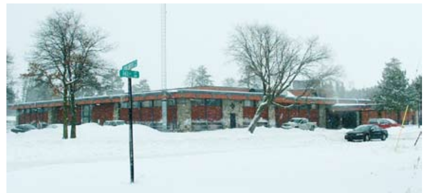
Cass Lake Facility Center built in the mid-1960's is in for a facelift. The Center will be remodeled and renovated to upgrade and meet building codes.
