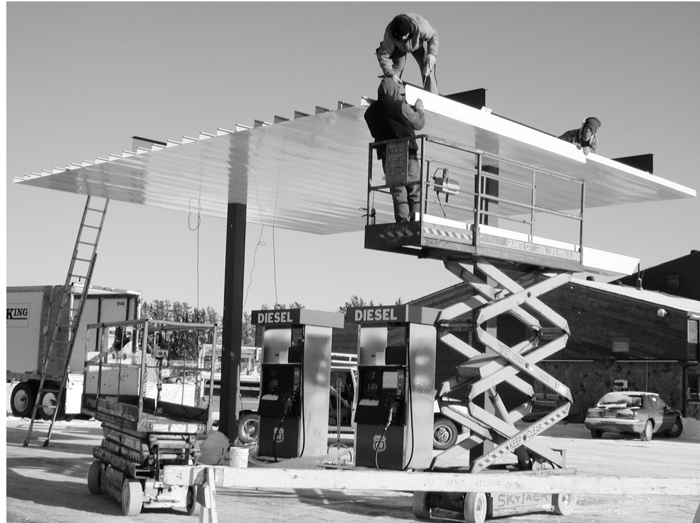
Che-We diesel pump receives a new camopy.
