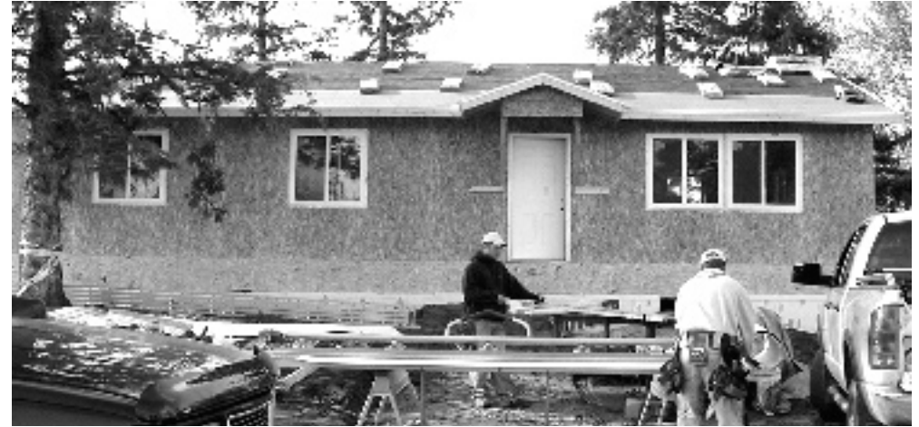
Model home currently under construction.
