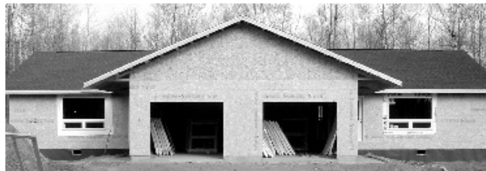
Duplex units under construction at Boy Lake.
