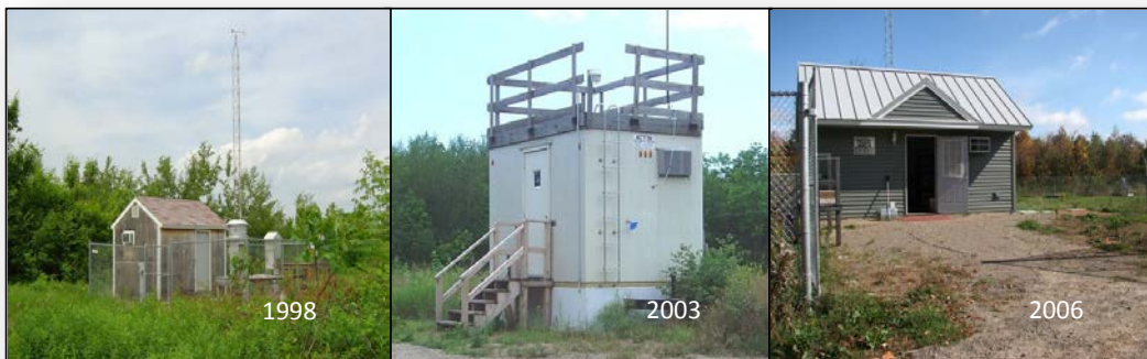
FCPC Air Monitoring Buildings
